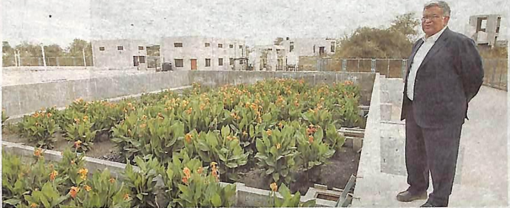
The plant is spread across 1,000 sqm. The system uses canna plants that are easily available in the city
